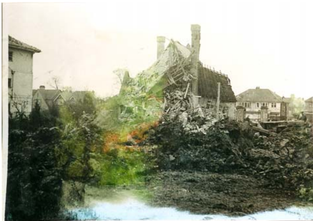
1940s photograph of the entrance lodge following bomb damage
