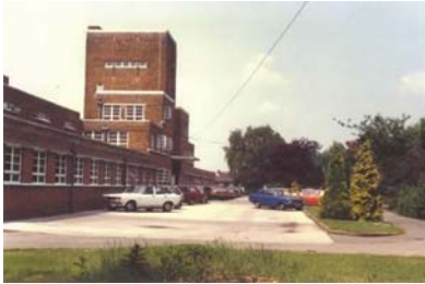
Historic photograph of the frontage
